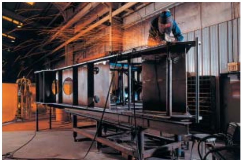
Final stages of welding the massive frame for the Darby 36" Series 2000 pipe bender.
